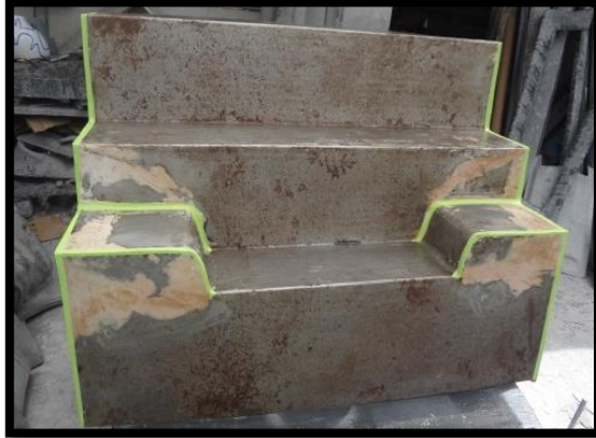
Figura 6-15 Colocar cinta masquin.
