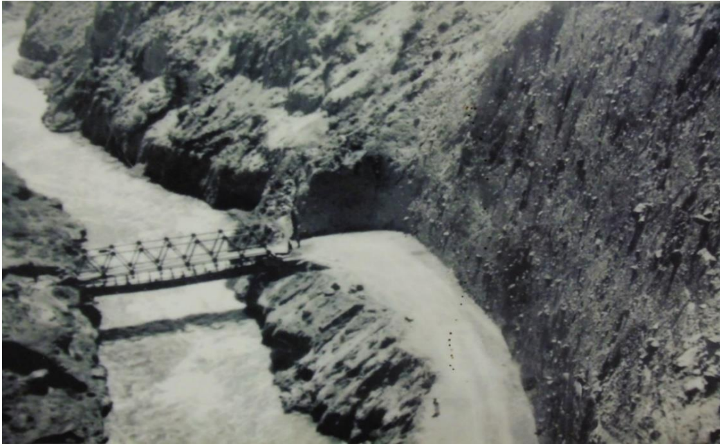
[Photo taken by: Alex Ramos] (Galo Plaza bridge,2017)
