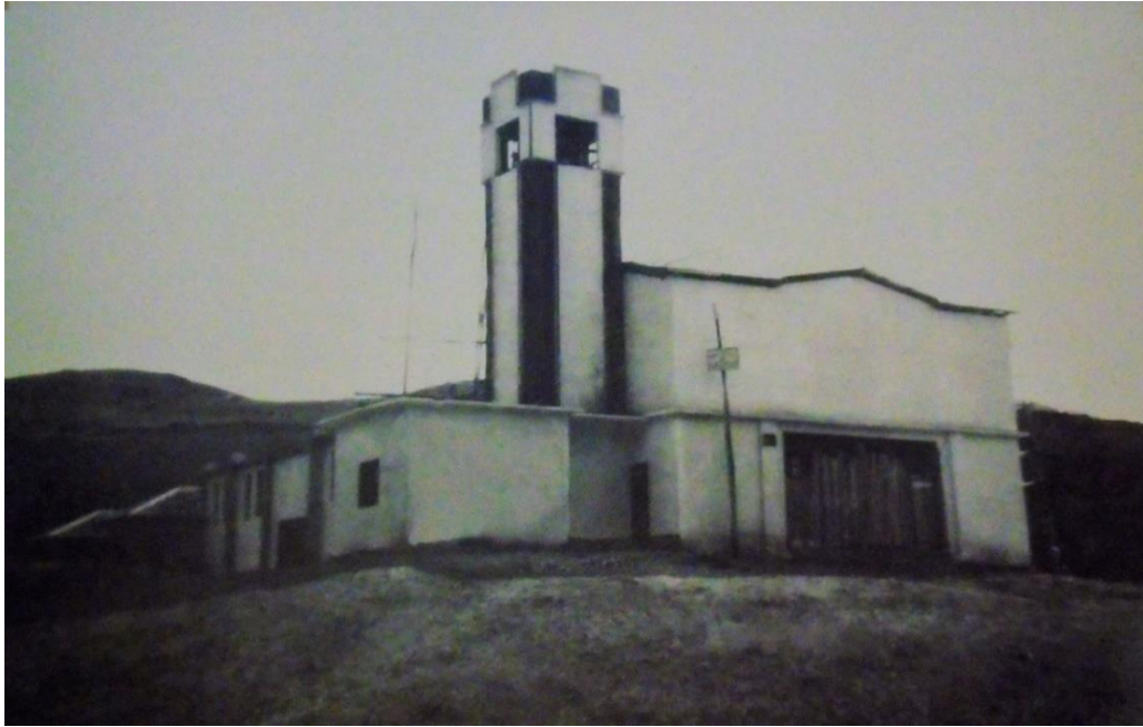
[Photo taken by: Alex Ramos] (New church in construction,2017)
