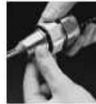
4. Slide armor stop insert over conductor and sealing compound, then back against armor. Pack remaining sealing compound.
