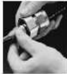
3. Mix sealing compound and pack conductors over armor.
