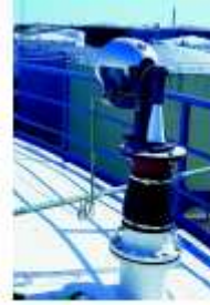
RTG 3940 is normally installed on the existing still-pipe when the tank is in service.
