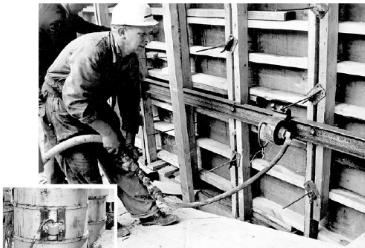
Fig. 6.5.3—Mounting of vibrators; wood wall form and pipe form (inset)
