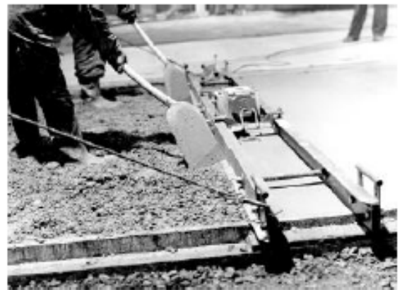
Fig. 5.4(b)—Vibrating screed for small jobs. Double beam type
