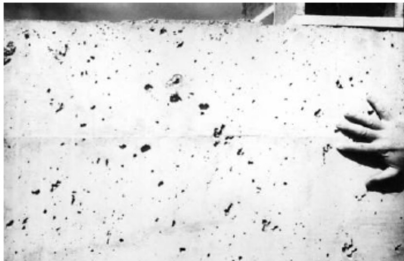
Fig. 7.6.2—Excessive air voids on formed surface
