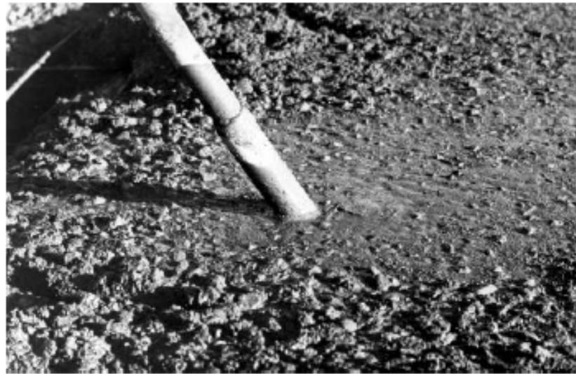
Fig. 4—Internal vibrator “liquefying” low-slump concrete
