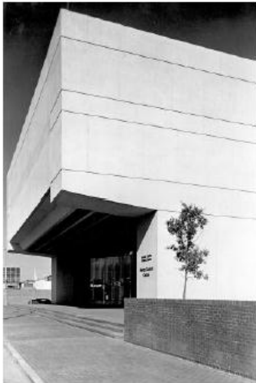
Fig. 1(b)—Pleasing appearance of concrete in utility building construction
