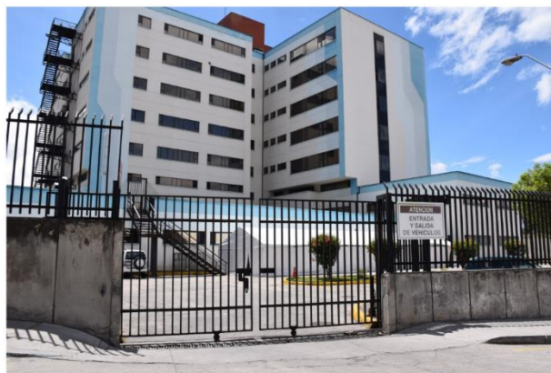
Figura 1.25. Hospital General Ambato IESS [42].
